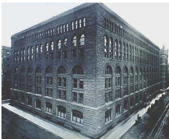
Figura 2: Club Warehouse (Chicago/EUA).
