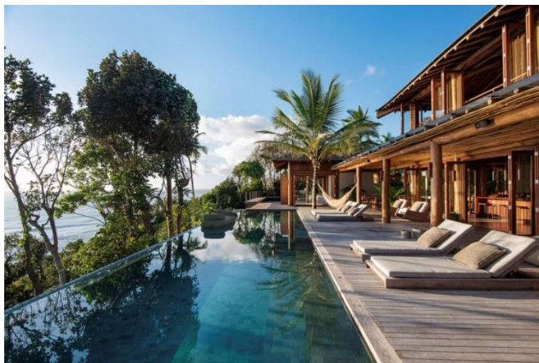
Figura 7 – Barracuda Hotel Boutique
